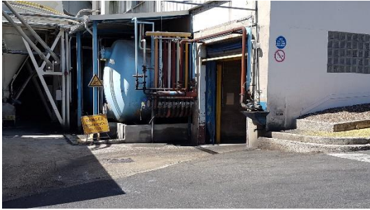
Installation Cuve 120B
